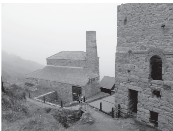
Rys. 5. Budynki kopalni Levant. Fot. autora Fig. 5. Levant Mine buildings. Authors photo
